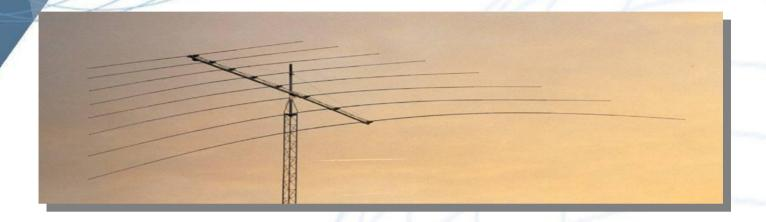
The RLP13-30 Log Periodic Dipole Array, is a highly directional HF antenna, operating in the frequency range 13 - 30MHz, designed for very long range HF voice and data communications.
